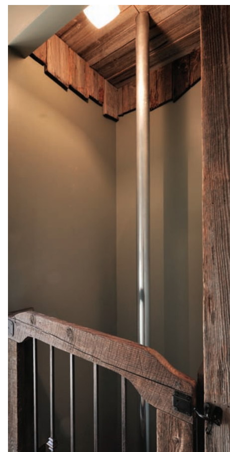
A gated 20-foot-tall firefighter's pole provides quick descent to the first floor.
